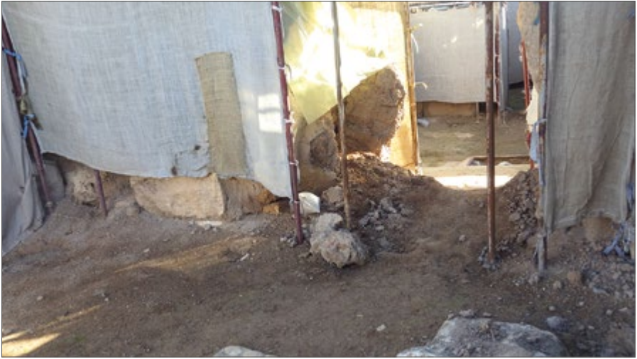
Fig. 5. Damage to doorway C5–C7 (January 3, 2017). This is one of two major losses suffered over the seven years of war (Courtesy IIMAS – The International Institute for Mesopotamian Area Studies)
