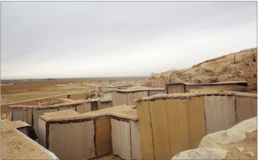
Fig. 6. Overall view of a sector of the Palace AP with old and new curtains (January 18, 2017) (Courtesy IIMAS – The International Institute for Mesopotamian Area Studies)
