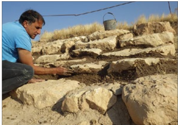
Fig. 2. Gaps between stones filled in with new mud, laid on top of a piece of burlap to keep it separate from the old mud (October 29, 2016) This process takes place in the fall, hence it was not done yet in 2017 (Courtesy IIMAS – The International Institute for Mesopotamian Area Studies)
