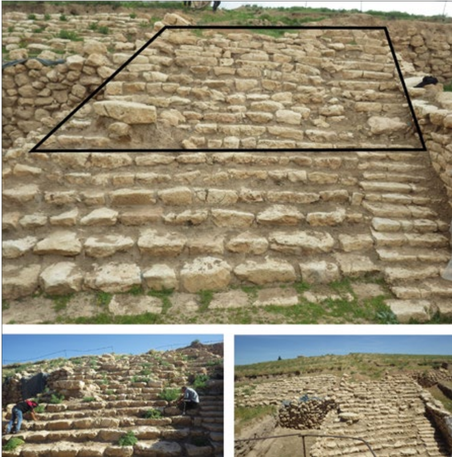
Fig. 1. Monumental staircase in Unit J2: top, after the first cleaning (March 27, 2017). It is interesting to note that the damaged portion of the staircase (in the black frame) is the result not of modern weathering, but of the disuse of the staircase in Mittani times, when the entire lower part of the staircase was covered by rapid accumulations. It is today the way it was first excavated in the 1990s; bottom left, during the second cleaning (May 5, 2017) and right, after second cleaning (May 7, 2017) (Courtesy IIMAS – The International Institute for Mesopotamian Area Studies)
