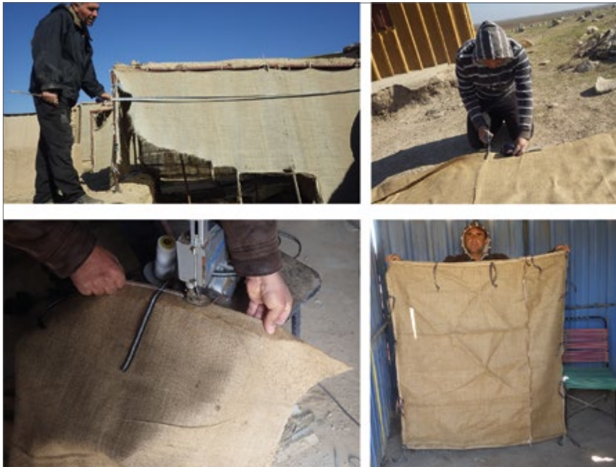
Fig. 4. New curtains being made: top left, taking measurements of a torn curtain to be replaced (January 12, 2017); top right, designing a new curtain (January 14, 2017); bottom left, sewing a new curtain (January 18, 2017); bottom right, a completed curtain before installation (February 2, 2017) (Courtesy IIMAS – The International Institute for Mesopotamian Area Studies)
